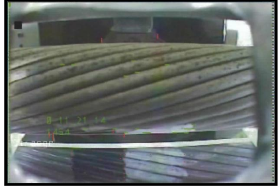
Figure 12. Sensors Placed around the Cables for Detailed Inspection of Surface Conditions [19]
